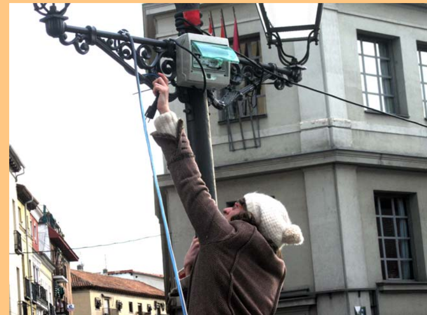
Maria repairs the electricity, December 2009 © Susanne Bosch
